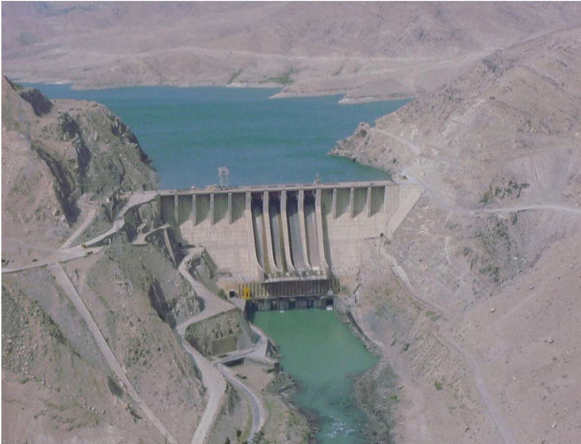
Figure 4. Naghlu hydropower dam [8].
