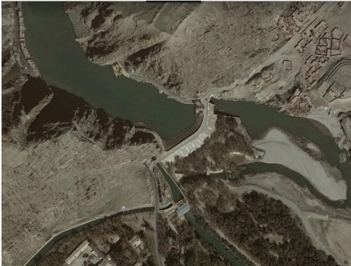
Figure 5. Darunta hydropower dam.
