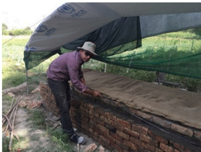
Figure 1. ZECC construction.
