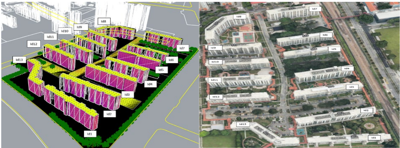
Figure 1. (a) Solar irradiance mapping – left (b) aerial view of Cheng San Crest with space ID of each HDB block – right.
